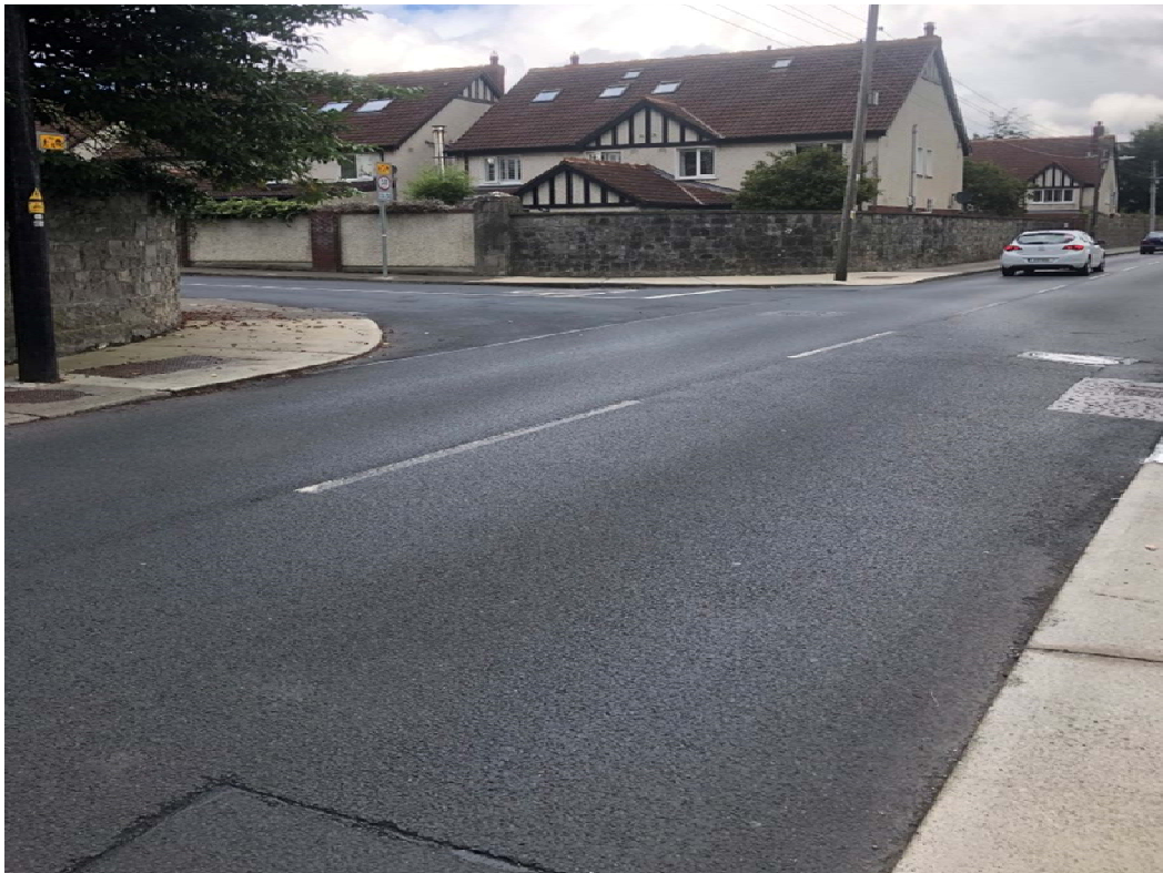
Figure 3-9: Existing Log Na gCapall-South Circular Road Junction-looking north east
