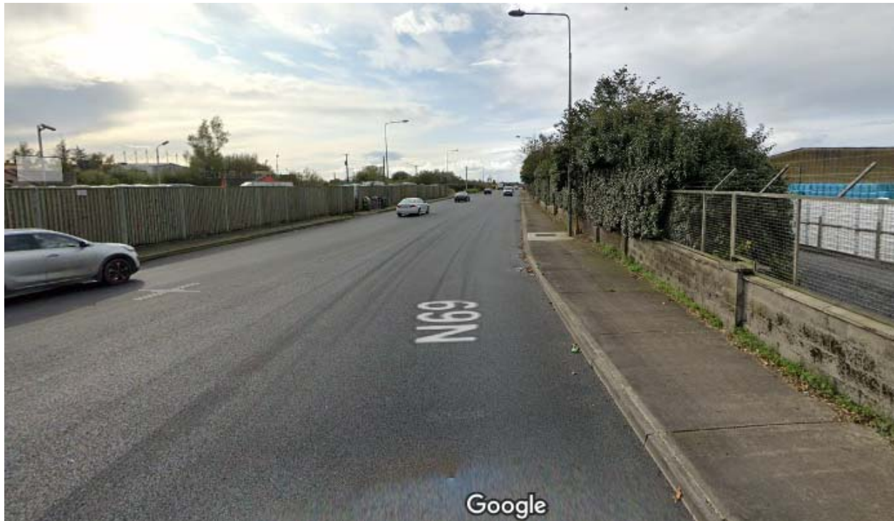
Figure 3-4: South west of Greenpark Roundabout-looking south west
