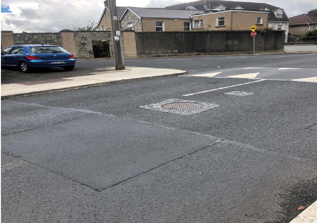
Figure 3-6: Existing Greenpark Ave-South Circular Road Junction - looking northeast
