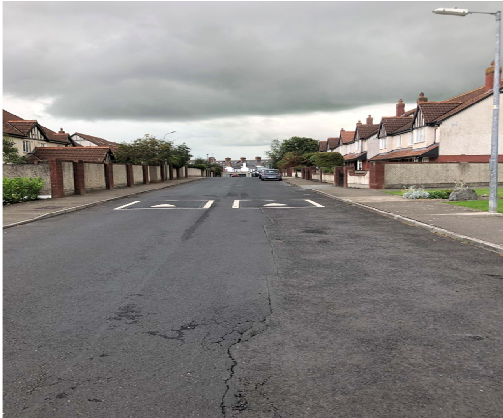
Figure 3-10: Log Na gCapall - looking northwest
